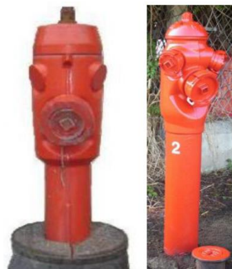
Figure 6 : Prise accessoire (PI DN80)
